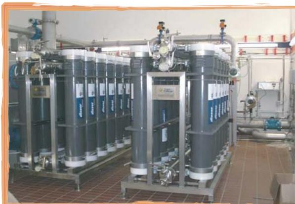
UF SYSTEM TO REMOVE COLLOIDS AND BOD
